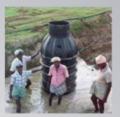
The strategically designed ribs on ASTRAL chambers interlock with the soil to prevent uplift. Engineering calculations show that DN 1000 ASTRAL chambers have a safety factor well over 1.8 against buoyancy caused by existing groundwater.
