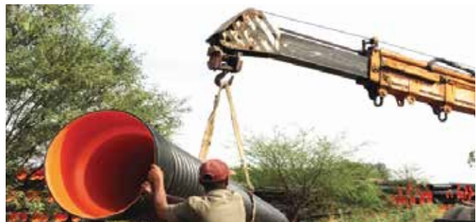
Handling of Pipes using Slings for Lifting
