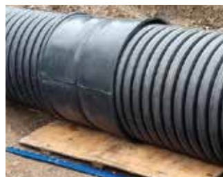
Figure 10: Example of Joint (Coupler Joint)
